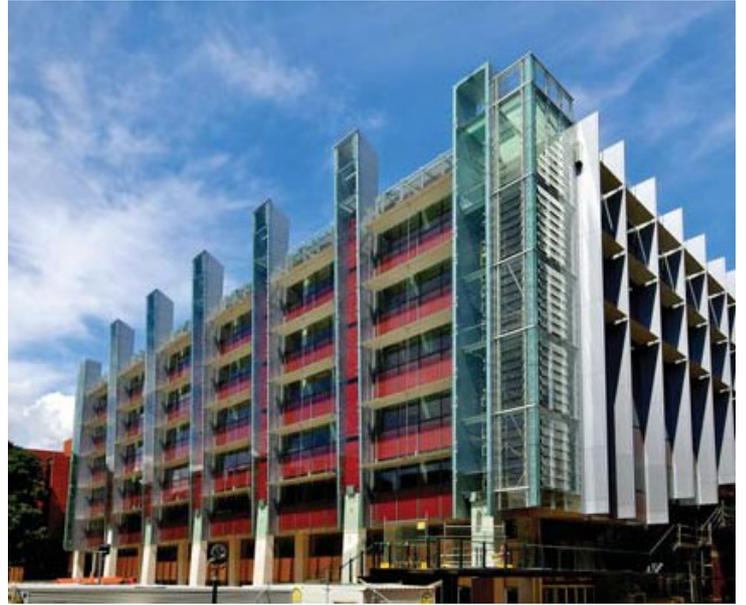
The recently constructed \$100 million Faculty of Engineering, Mathematical and Computer Sciences building, Innova21, has a six star rating for environmentally sustainable design. The architects and engineers have included solar photovoltaic panels on the roof to provide 2kW of renewable power to the building. There is an extensive rainwater harvesting system of 500,000 litres capacity that supplies water for flushing the toilets and any internal irrigation.
